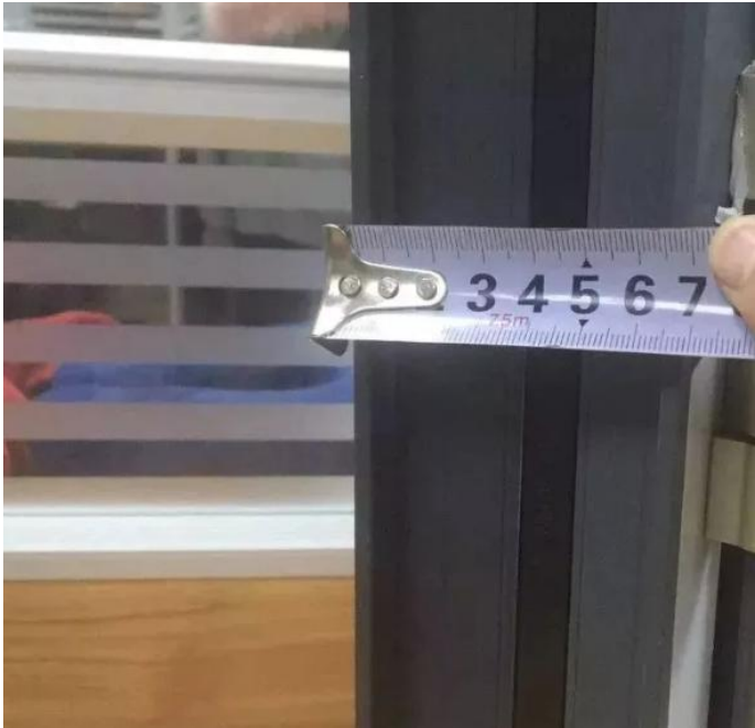
▲70 型材，指窗框含隔热条宽 70mm
